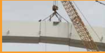
Moses Mabhida Stadium - Pfizer Germany - Lifting and Installation of Main Arch
